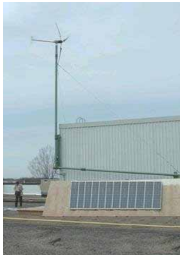
The CDDHS Wind Turbine and Solar Panels, on the school roof
